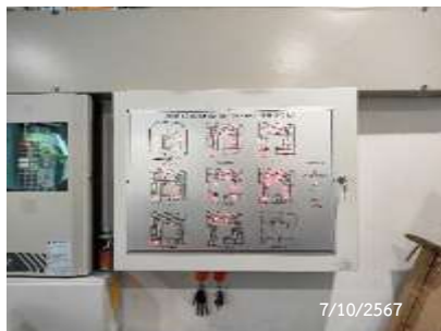
Graphic Annunciator Fire Alarm System
